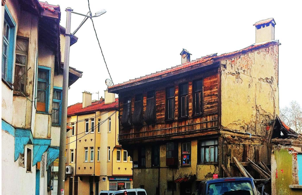
Figure 2. Buttress and outbuildings wooden houses (writer archive,2014)
